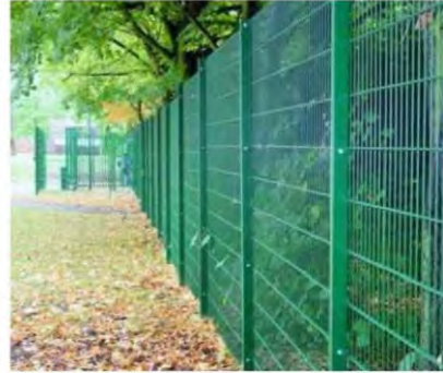
Reference image - 1.8m High Weldmesh fencing
